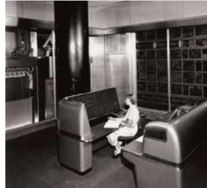
*IBM’s SSEC super calculator pointed up a critical problem: electro-mechanical input, output, and memory sources could not keep up with the new computing speeds.*
